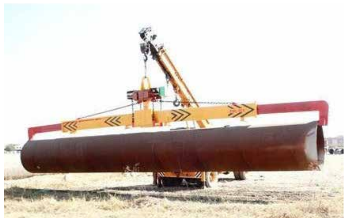
Pipe Lifting Tackle
